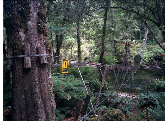
A bridge with low capacity
