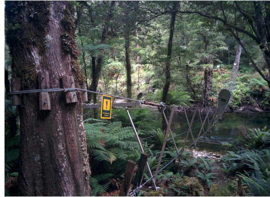
A bridge with low capacity
